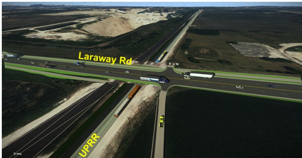
Figure 21a: UPRR under Laraway Road with Common Design Characteristics
